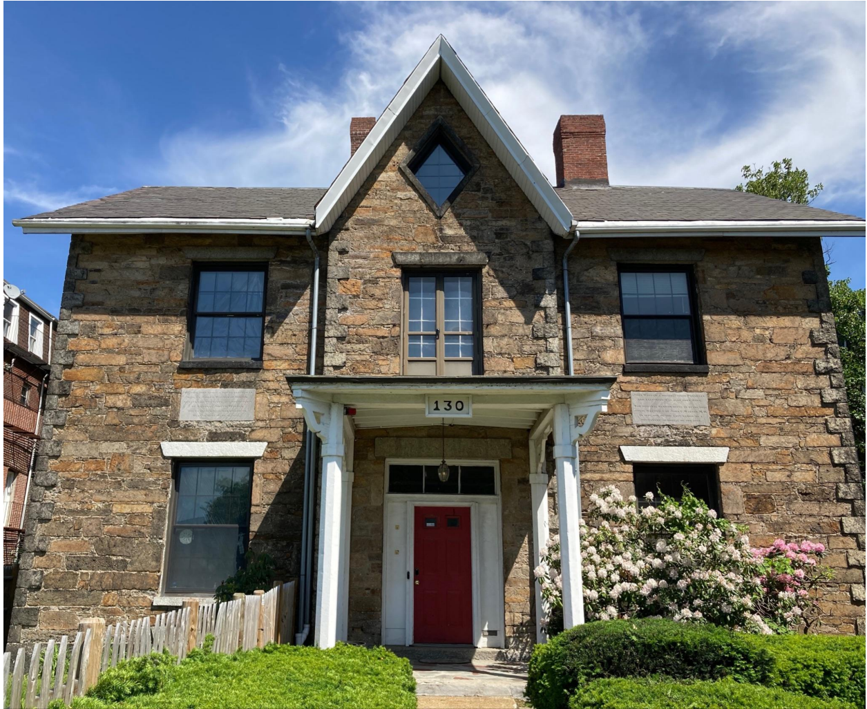
Figure 2: Entrance Front facade (west elevation)
