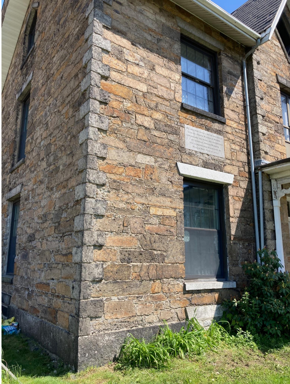
Figure 6: Quoins detail Corner between the west- and north-facing facades
