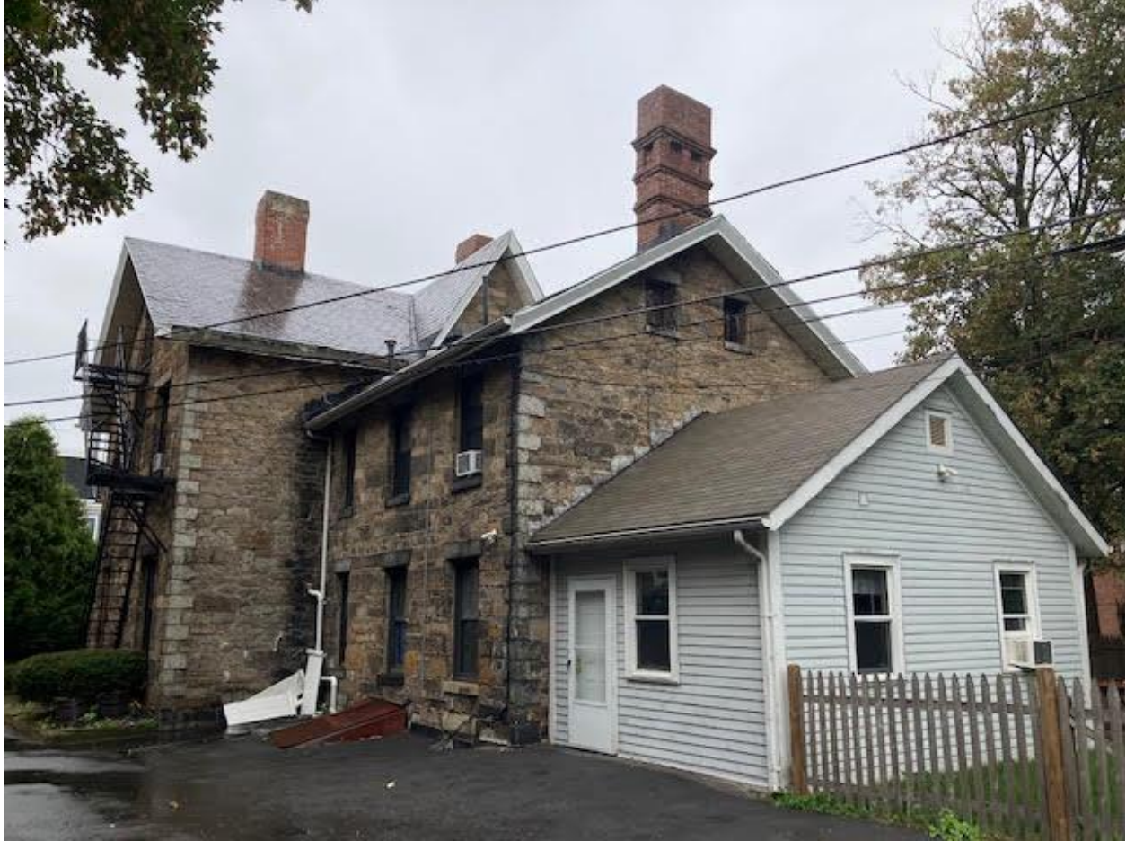
Figure 11: Rear of building (southeast corner)
