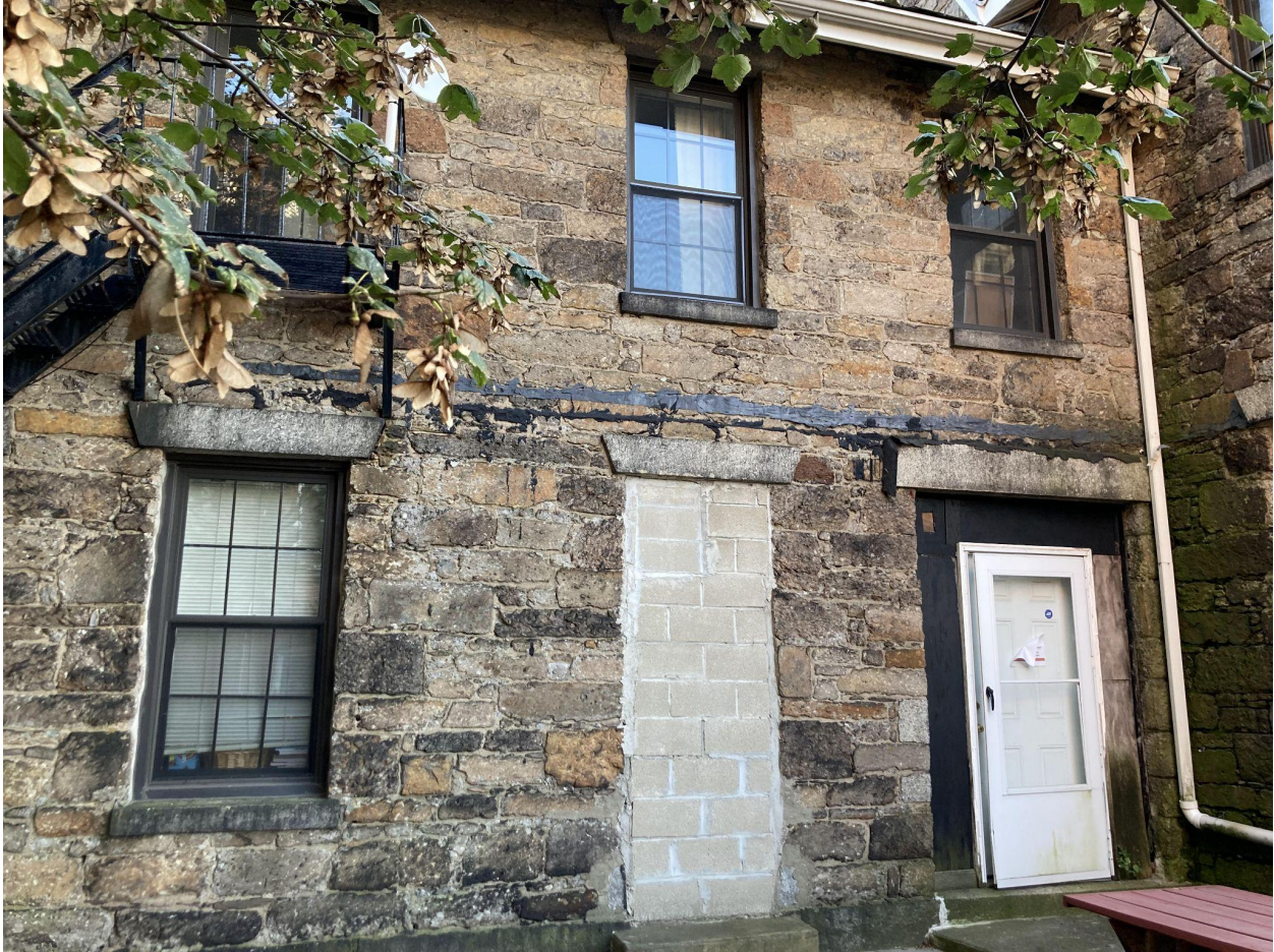
Figure 16: Closer look at the north elevation of the rear wing
